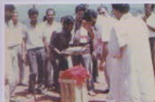
Sjt. Atul Bora Former P.W.D. Minister laying the foundation stone of our 1st Building on 6th May, 1990
